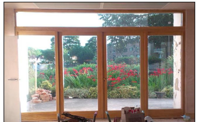
Almost finished! Looking through the new, transparent doors
